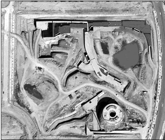
Fig. 12. Site photo of previous state of the Emergency Hospital in Madrid [material from Cristina Jorge archive]
