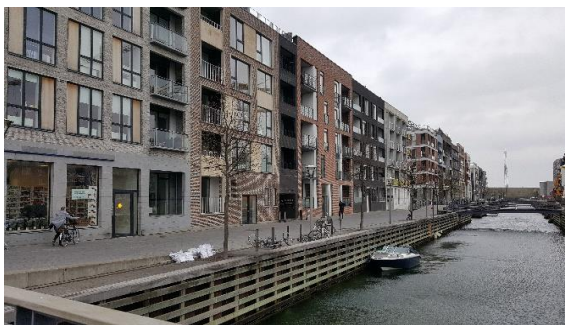
Fig. 4. Sluseholmen canal infrastructure [photo Una Īle, 2018]
