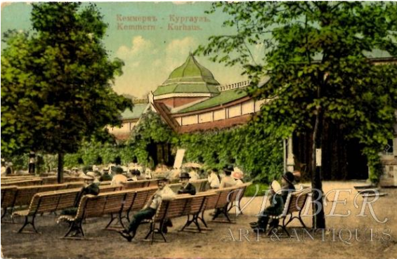
Fig. 15. Walls with climbing plants near the stage, the early the 20 th century. NJKP archive.
