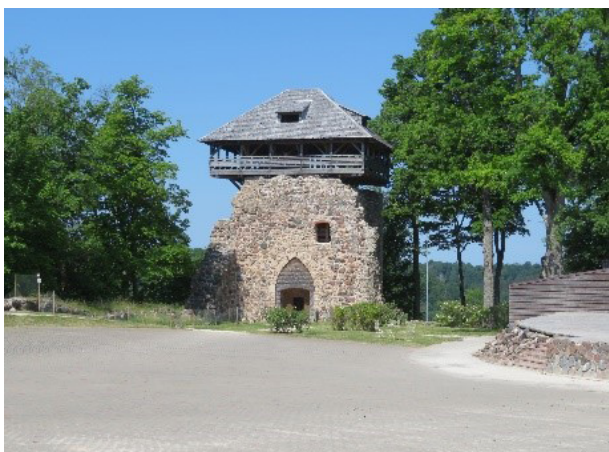
Fig. 13. Conservation structure of the watchtower as a tourist viewing platform at Sigulda Castle ruins [photo by O. Spārtiis]
