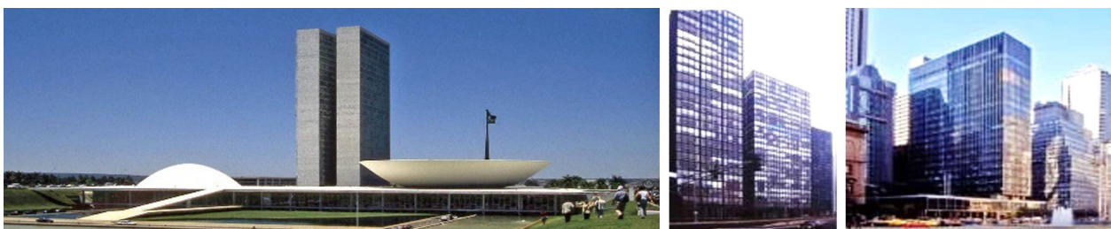
Fig. 41. Brasília, Brazil. Congress Palace. 1959–1960. Oscar Niemeyer Fig. 42. Chicago, USA. Residential buildings at 860–880 Lake Shore Drive. 1948–1951. Ludwig Mies van der Rohe Fig. 43. New York, USA. Lever House at 390 Park Avenue. 1952. Gordon Bunshaft
