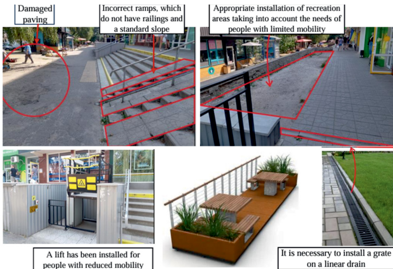
Fig. 3. Problem areas at the entrance to shops located on the first floor of a residential building built during the Soviet period, Poltava (Ukraine). Author – Natalia Novoselchuk. [from N. Novoselchuk scheme]
