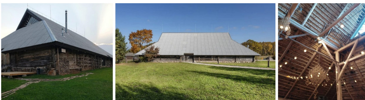
Fig. 5. Barn transformed into a party hall with a professional kitchen (architect - Mantas Maziliauskas), Pagulbis village, Molėtai district municipality. Photographs by I. Raudnikytė and L. Garbačas
