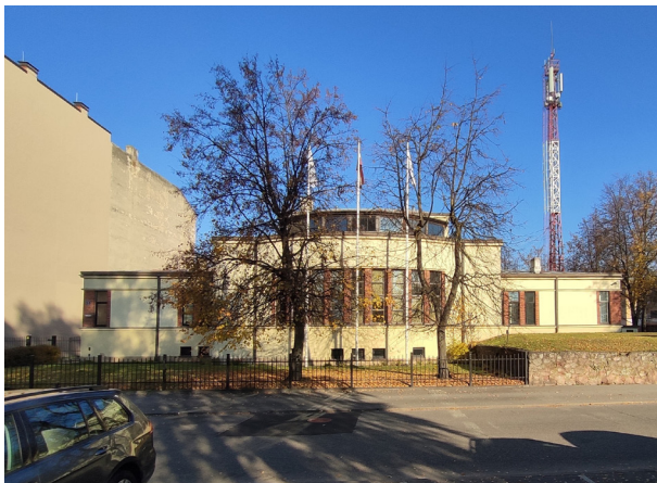
Fig. 17. Transformer substation at Stadona iela 1. Architect Artūrs Ramanis. 1939
