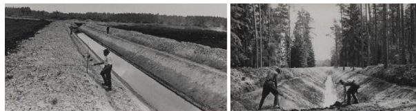
Fig. 8. Victory Pike. Establishment of a ditch system for clearing fields in the 1930s 20th century Fig. 9. Victory Pike. Ditching through the forest in the 1930s
