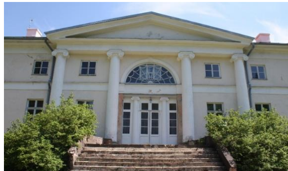
Fig. 6. The central portico of the manor house [photo by author, 2014]
