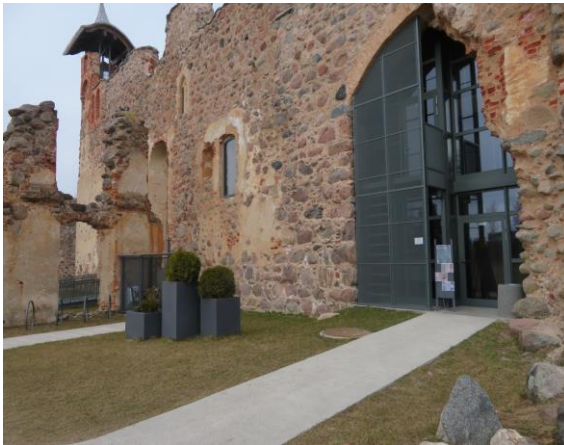
Fig. 5. Steel-and-glass construction as replacement of the ruined wall [photo by the author]
