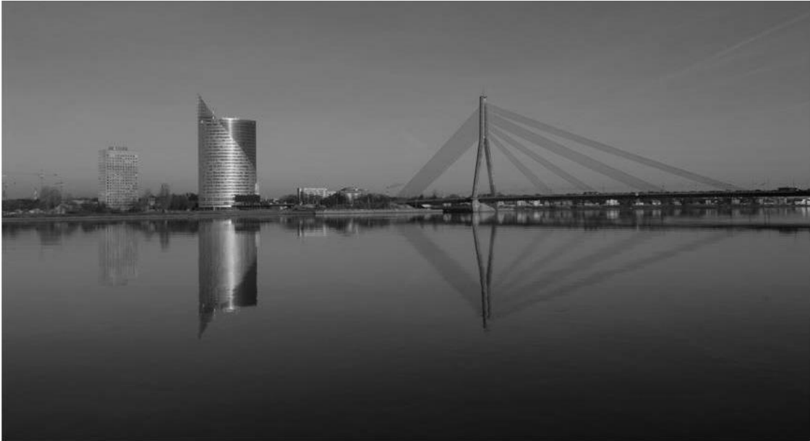
Fig. 3. The housing on the left shore of the Daugava River near the Vanšu tilts (Cable-stayed Bridge) [Source: photo by J. Krastiņš]
