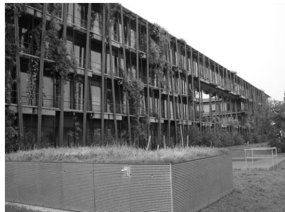
Fig. 5. Possibilities to introduce the containers with the plants in the structure of building facade. Walter Nernst-Haus, Institute of Chemistry, Humboldt University, Adlershof, Berlin, Germany [Source: photo by the author]
