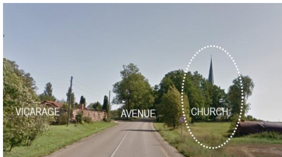
Fig. 7. The overgrown trees obscure the elegance of the church. Kabile church, 2021 [the authors' photo]
