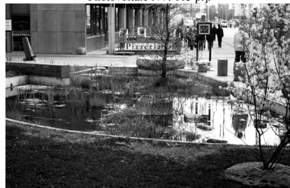
Fig. 17. A concreted pool with aquatic plants accumulates rain water during the rain, Malmö, Sweden [Source: photo from K. Siļķe private archive].
