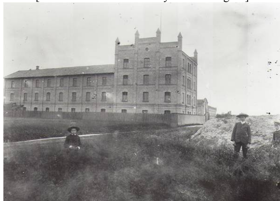
Fig. 11. Palīdzības street. The prison building, the beginning of the 20 th century [Source: Museum of History and Art Jelgava].
