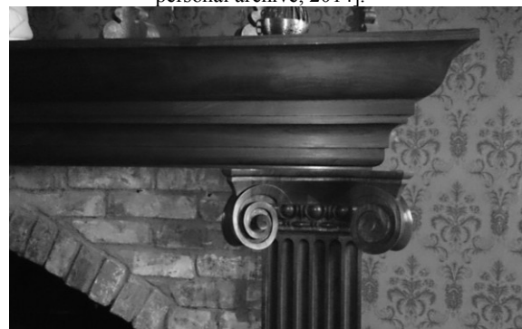
Fig. 4. Fragment of the mantelpiece of the Brukna Manor dining-hall [Source: photo by author Aija Grietēna personal archive, 13.04.2014].
