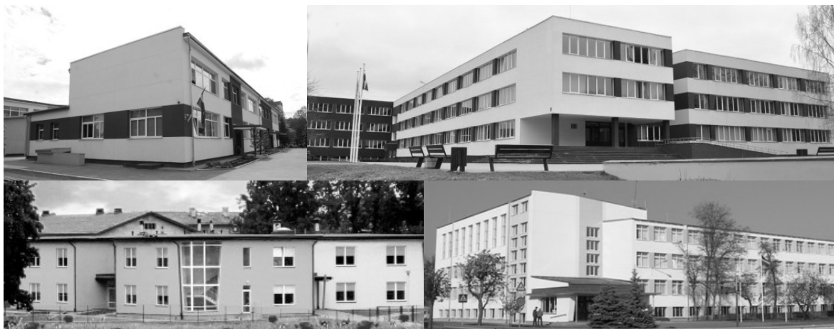
Fig. 7. Insulated buildings in Olaine with finishing in different colors [Source: from the Olaines municipality webpage: http://www.olaine.lv/izglitiba ].
