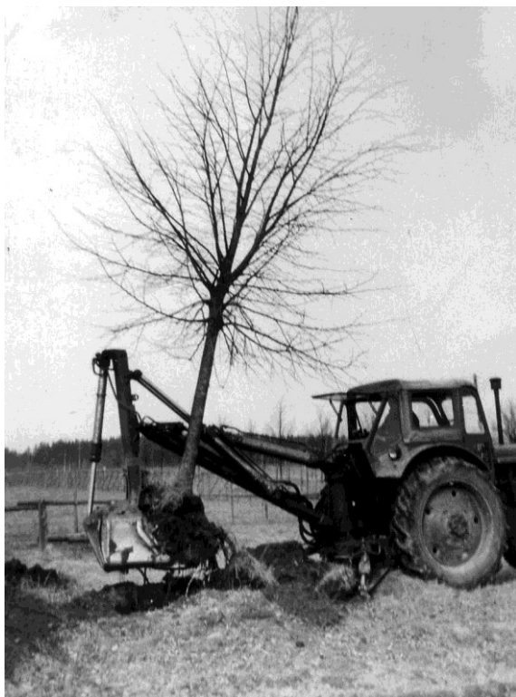
Fig. 4. Digging out trees from alleés, 1970 [Source: Latvian road museum].
