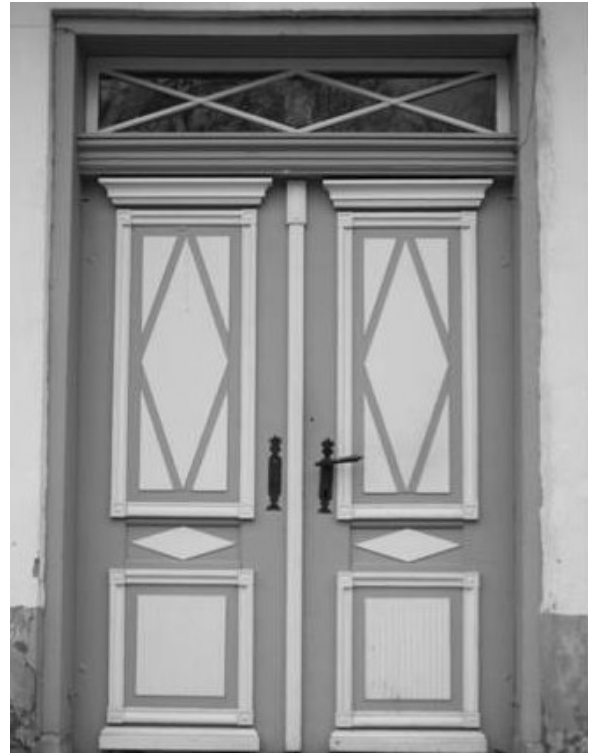
Fig. 7. The main entrance door leaves of the rectory [Source: photo by author, 2013].
