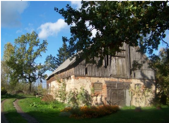
Fig. 8. Clay molding with stone joining elements in the corners. Jaunsvirlaukas Parish [Source: photo by author, 2013]
