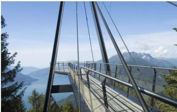
Fig. 20. A part of the Cardada project - The viewing platform. [Source: http://jakem.ch/html/bruecken_en.php ]
