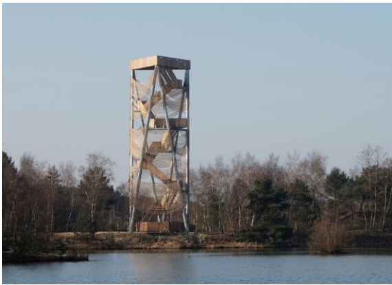
Fig. 1. The Lommel observation tower [Source: http://www.archdaily.com ]
