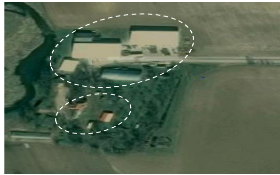
Fig. 18. Nearby the individual farmstead of the new farm, the agricultural production of the start of the 21 st century has grown with an exaggerated scale of buildings and roads, Jaunsvirlauka Parish [Source: author scheme and google material, 2016]
