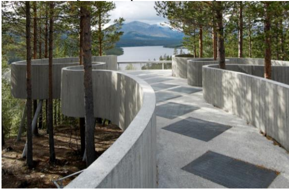
Fig. 14. The Sohlbergplassen observation deck [Source: http://www.archdaily.com ]
