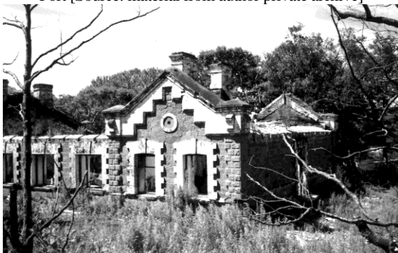
Fig. 11. A barrack (Russky Island) [Source: material from author private archive]
