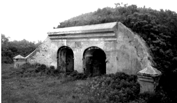
Fig. 10. A caaponier for withdrawable guns in the Pospelov 2 Fort [Source: material from author private archive]
