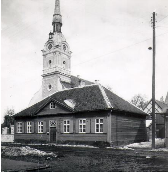
Fig. 4. The former Reformed Church on Uzvaras street [Source: JHAM]
