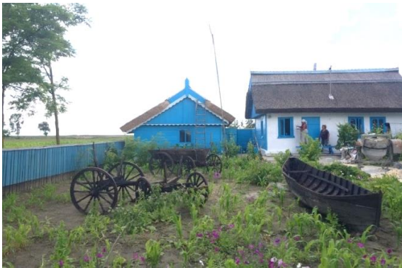
Fig. 4. Preserving the vernacular architecture of Danube Delta and the sensible relationship with its natural and cultural landscape in the development of touristic facilities [photo: M. Sbarcea]
