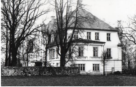
Fig. 13. View of the Malpils Manor. Photo of the 1990s [NKMP PDC]
