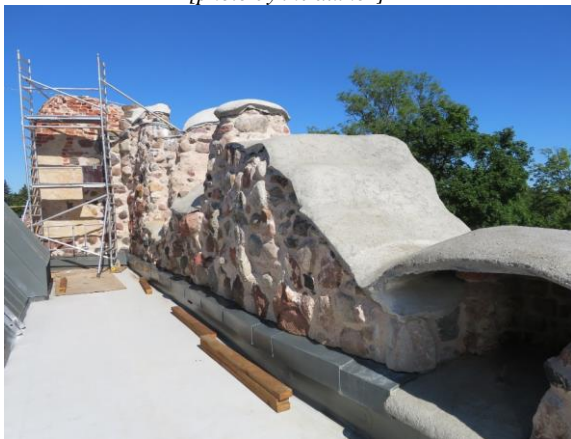
Fig. 10. Coverage of the upper part of walls with fibro-concrete [photo by the author]
