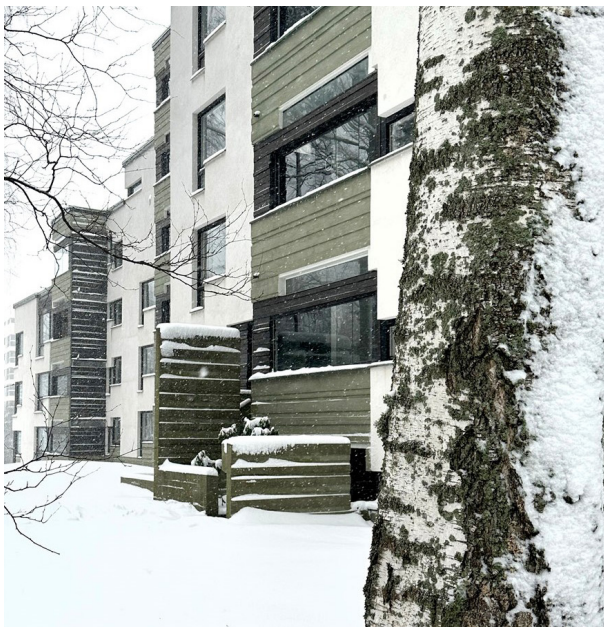
Fig. 9. Photograph of the Suvikumpu residential complex, 2023 [the authors]
